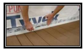
Install or reinstall siding if it has been removed for the deck installation. Install waterproofing butyl tape to the deck board (7/8") and deck post at all locations where a "through the deck support post" penetrates the deck to assure that water does not find its way through the deck to the area below.
