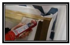
If the length of the board will be placed along a wall of the house also place a bead of sealant on the joist where the board will rest.
