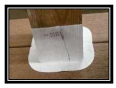
The waterproofing butyl tape will be concealed by the post sleeve and base trim when the rail system is installed.
