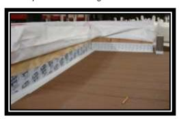
Turn the house wrap material down over the flashing and seal the house wrap material to the flashing with a sealing tape.
