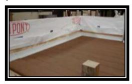
Seal the flashing to the wall under the house wrap using a sealing tape to assure that any moisture that penetrates the house wrap will not find its way behind the flashing.
