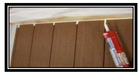
Cut and position coated aluminum (or other material) flashing with the flashing being install behind the house wrap material and over the decking.
