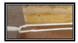
Move the flashing into position behind the house wrap material and over the decking assuring that the sealant is bonded to the decking and flashing.
